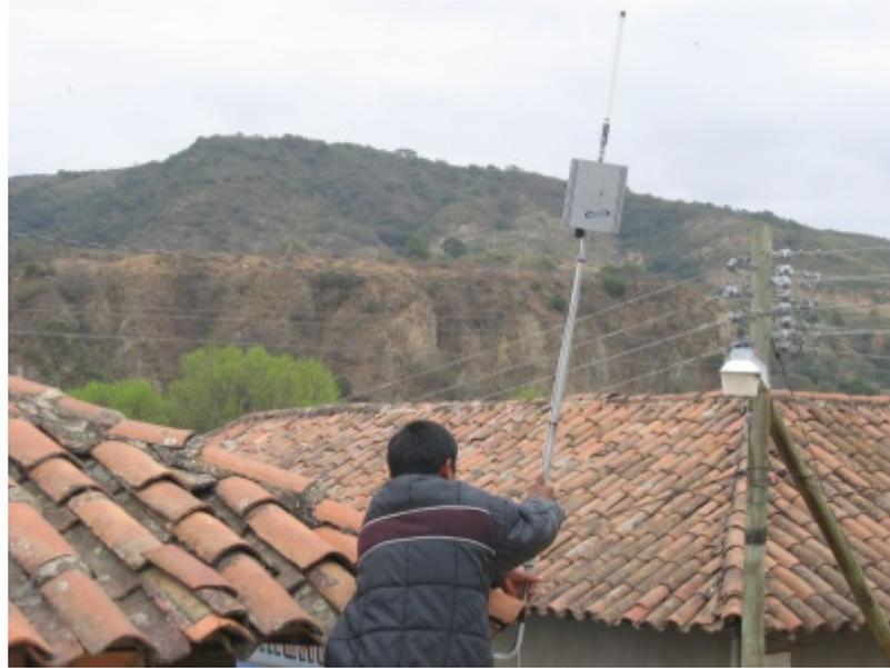
Figure 18 Locust World mesh box installation in Bolivia
